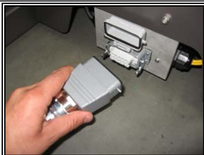
Left – Plugging in Quick Disconnect
